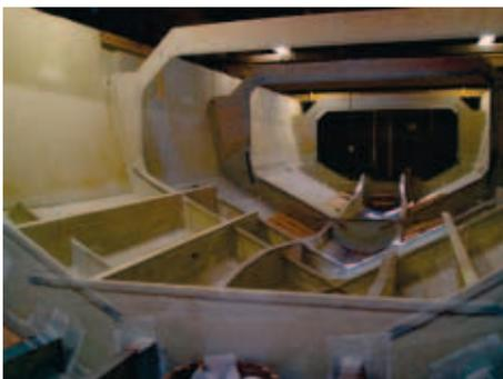
Figure 3: Partial bulkhead Installation
