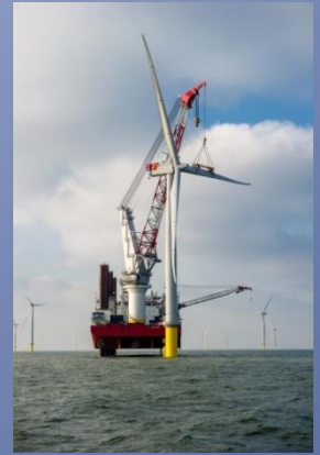
Copyright: London Array Ltd.
