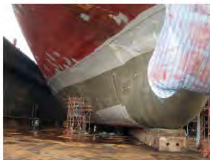
Masking of surrounding areas during FRC application
