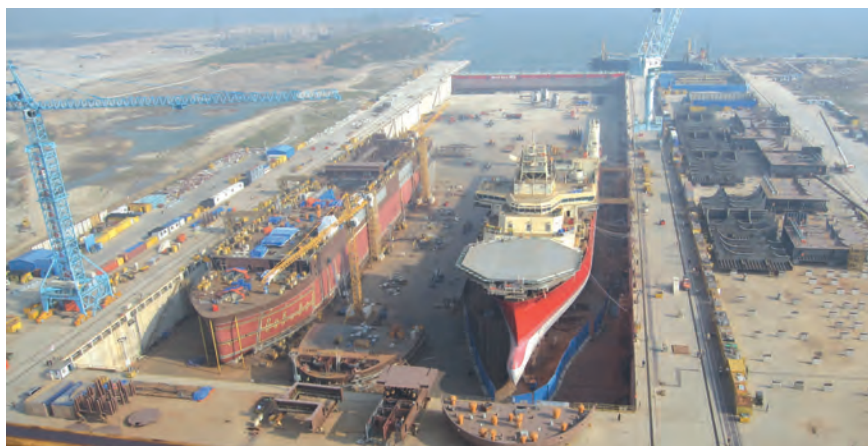
STX Dalian's Changxing Island site covers an area of over 5.5 million m 2 , and can lay claim to being the largest shipyard in the world
