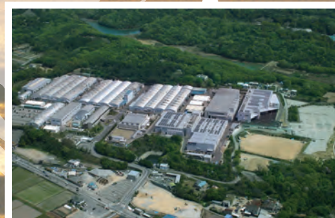
Kawasaki Heavy Industries, Ltd. Nishi-Kobe Works
