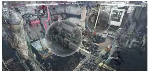
ENGINE ROOM THE USE OF SCANNING TO INSPECT EQUIPMENT AND MEP
