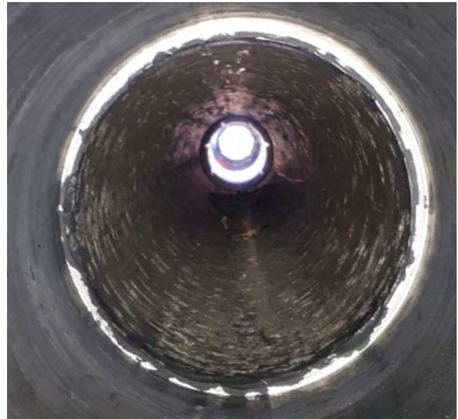
Figure 4 – Belzona bearing housing recess restoration
