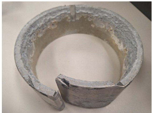
Figure 2 – Mid Sacrificial Sleeve Insert removed after 10 months of installation
