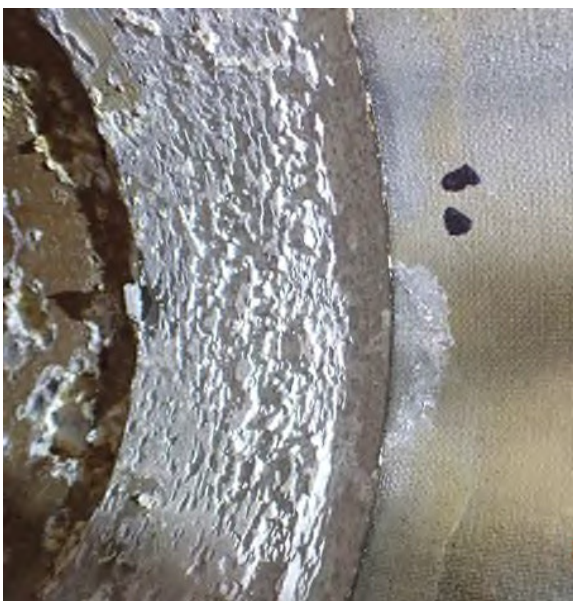
Figure 18 – Port Fwd Location 2 (3 O'clock) Corrosion 6M
