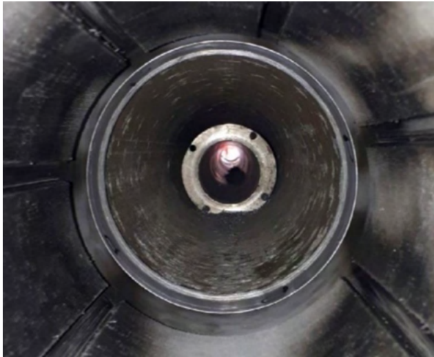
Figure 13 – New Aluminium Sleeve Installation - (Typical Port and Stbd)
