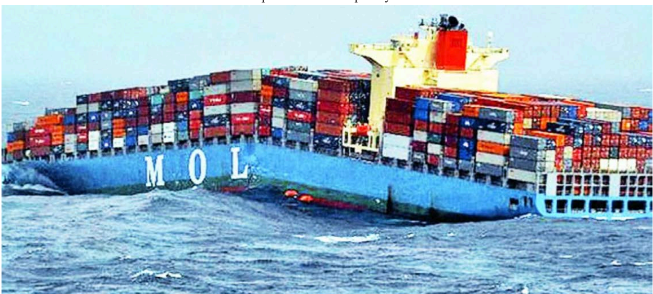
Figure 2: Buckled MOL Comfort before separation of hull sections (Photo from Core77 website)
