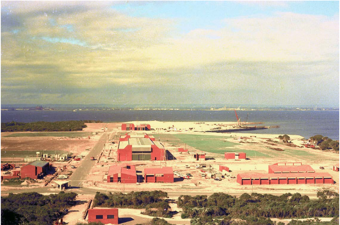
Construction of wharves and workshops for the new naval base began in early 1973. Work was well advanced by the time this view of the site was taken in August 1974. The base was commissioned as HMAS Stirling on 28 July 1978 (Photo John Jeremy)
