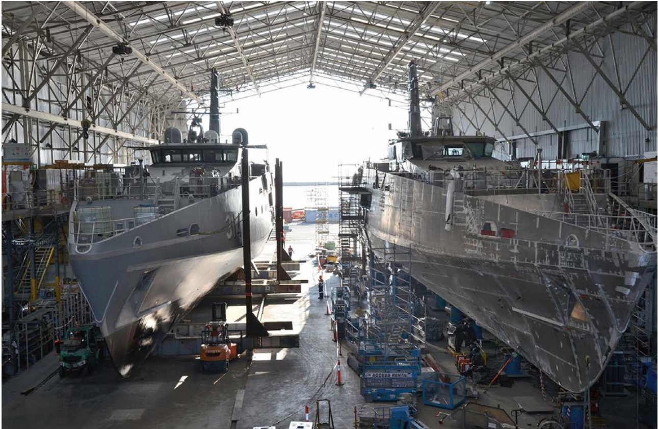
Two Evolved Cape-class patrol boats under construction at Austal's facility in Henderson, Western Australia (Photo courtesy Austal)
