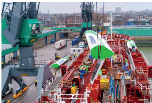
INSTALLATION OF THE VENTOFOILS. SOURCE: CHEMSHIP
