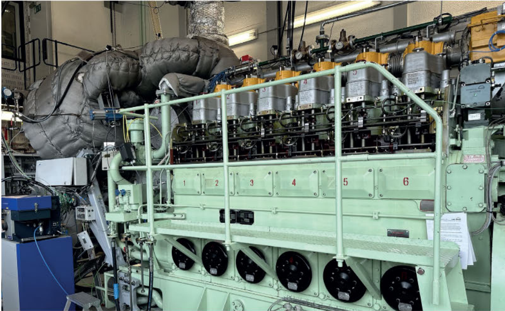
TOWARDS AN OXICAT-EQUIPPED FOUR-STROKE: TEST ENGINE RUNNING UNDER THE IMOKAT II PROJECT. SOURCE: MAN ES
