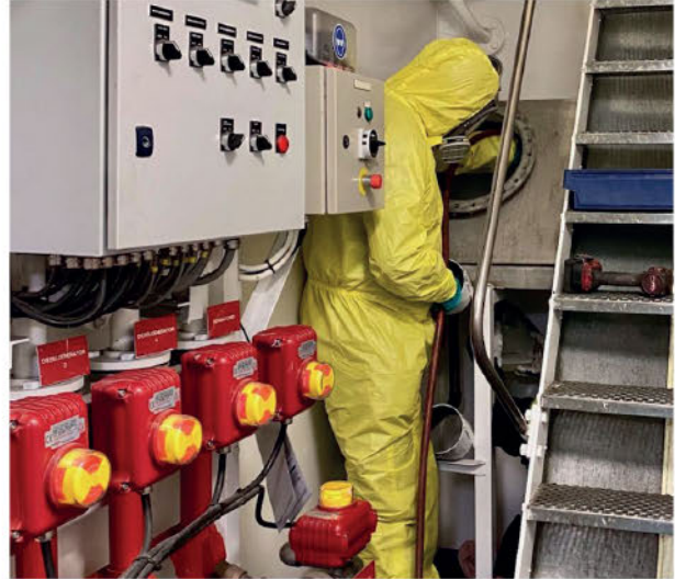
TANK INSPECTION AFTER DECONTAMINATION. SOURCE: SCANUNIT
